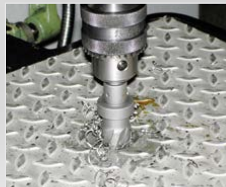
Drilling structured sheet metals
